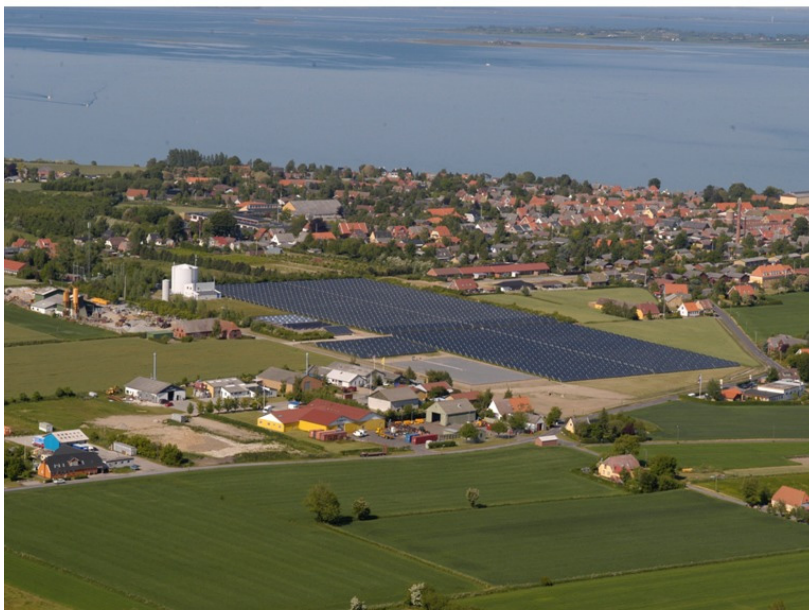
Figure 19. View of the Marstal solar collector area in Denmark. Photo by permission from Leo Holm, Marstal Fjernvarme.
