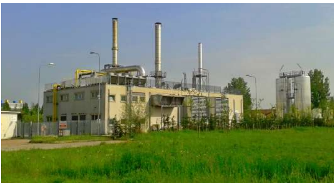
The CHP / DH Plant after the modernization, with Thermal Energy Storage on the right
