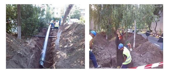
4. The speed of installation of the pre- insulated PB pipes, 3 to 4 times faster than classical systems, greatly
