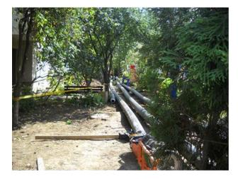
2. The elasticity of the pre-insulated PB pipes also permitted the evasion of trees, manholes and other obstacles (which greatly reduced the impact on green spaces). They have also permitted the passing of 30 up to 70m sections under other networks: methane gas, drinkable water; sewage; electricity cables; telecommunication cables etc, through their curving and sliding on a 10 cm sand layer.
