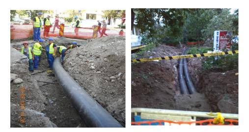
6. It was also possible to avoid affecting some alleys, streets, parking spaces and green spaces through the use of the old concrete ducts created in the 80's for the transportation of geothermal water, through which 70m sections have been slid through a very narrow space. The sections slid on a concrete tile base of the ducts that had a width of merely 60 cm, the two sections of pre-insulated pipes both having an external diameter of 250 mm, totaling 50cm.
