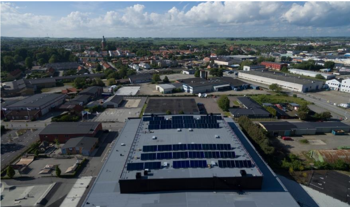
Figure 55: Feed-in solar heating system on the sports arena in Ystad.
