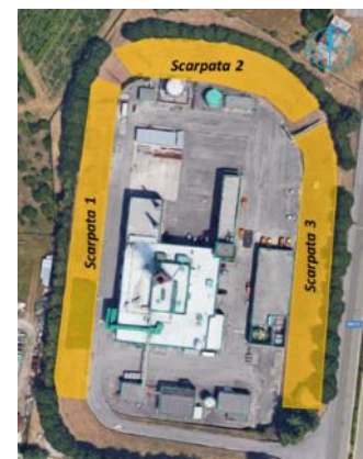
Figure 30: Verona: Slopes around the heating plant
